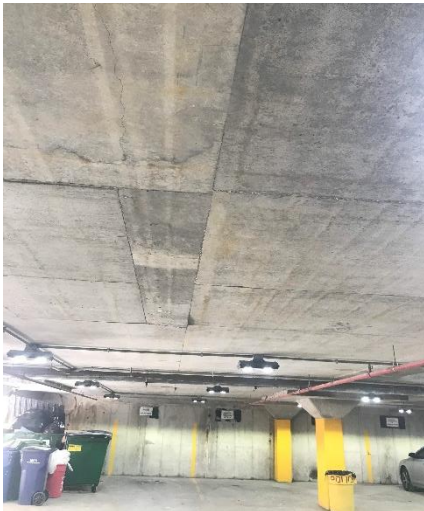
Repaired concrete deck at garage
