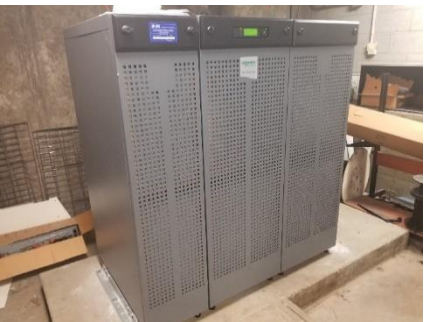
UPS battery back-up system
