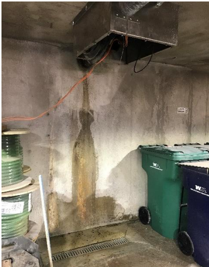
Water infiltration at pipe penetration
