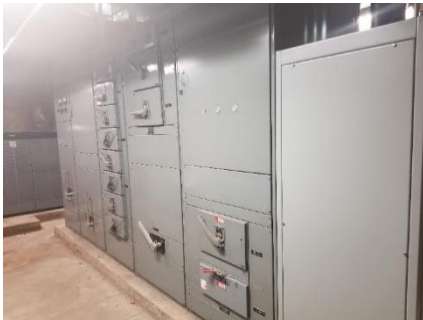
Main electric service switchboard
