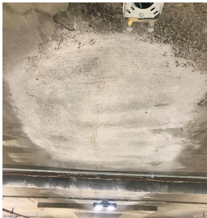
Area of patched concrete deck at garage
