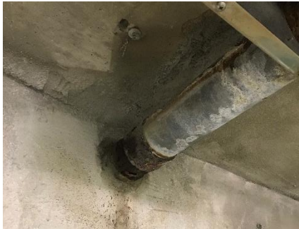
Repaired conduit within garage
