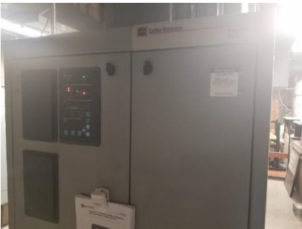
Main emergency transfer switch
