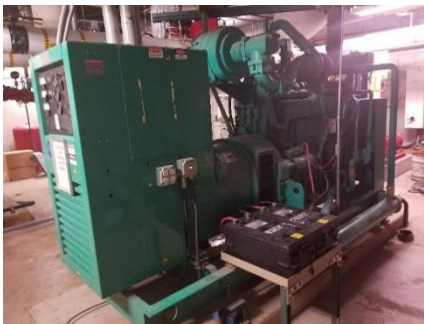
Main gas-fired back-up generator set
