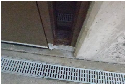
Steel door frame is corroding
