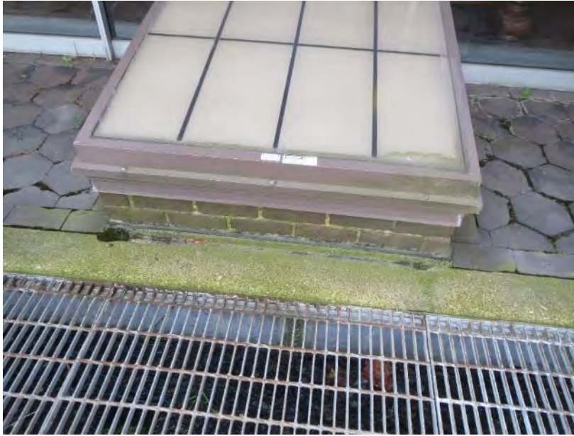
Figure 58. Sealant has been smeared over the face of the skylight. Debonded sealant in the joint between the concrete curb and the base of the skylight. Note displacement of pavers and organic growth at pavers at skylight.
