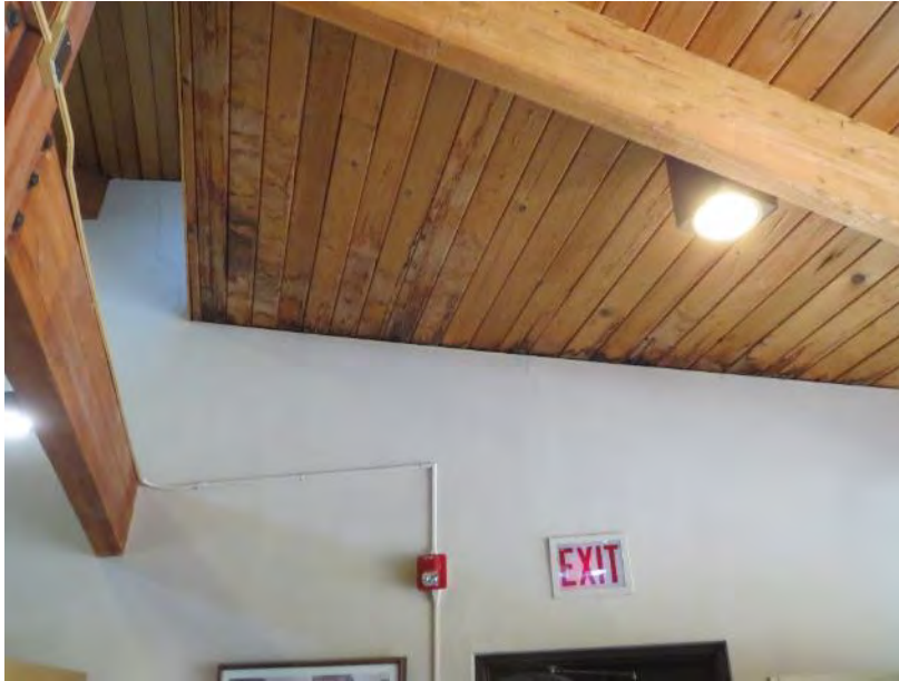
Figure 64. Water staining at the wood deck above the drywall at the east wall at the north portion of the building. This is coincident with a location of previous leaks.
