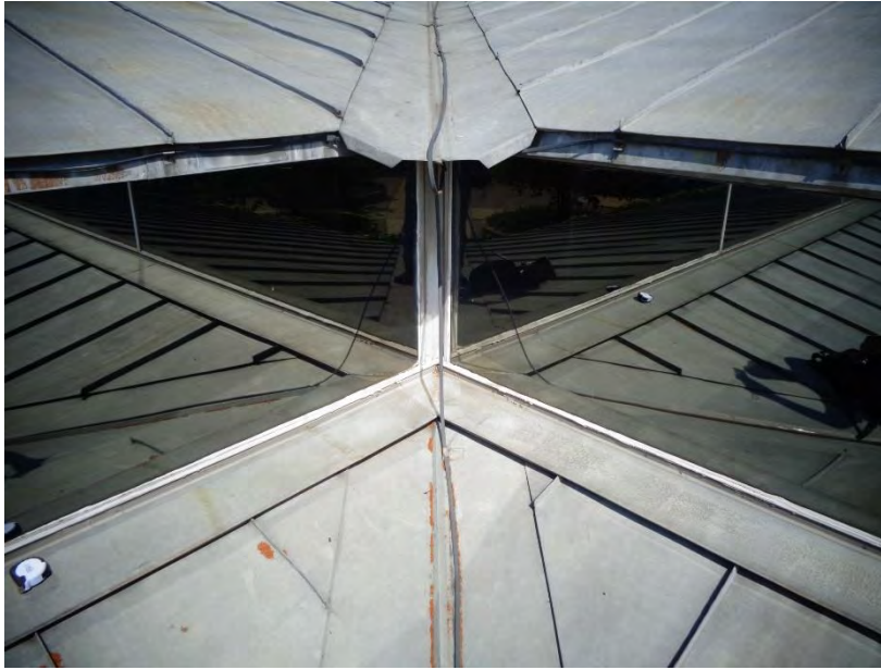
Figure 72. View of valley configuration at lower and upper low slope roofs
