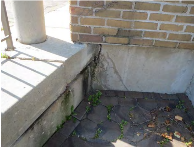
Figure 33. Crack at concrete foundation wall at the intersection of the base of the ramp
