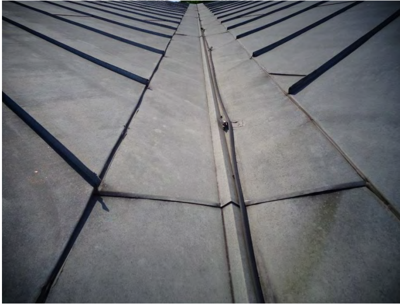
Figure 82. Close-up of sheet metal valley
