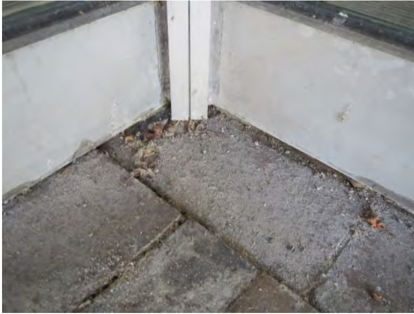
Figure 54. Missing sealant in the joint between base of window wall and pavers
