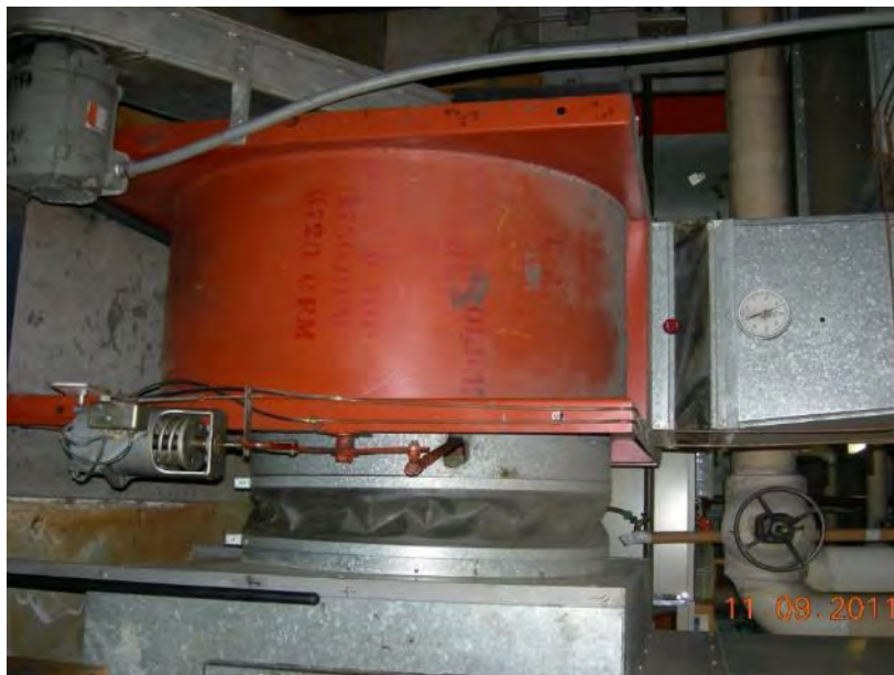
Figure 144. Typical pneumatic actuated return/exhaust fan damper
