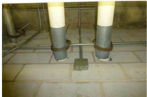
Figure 110. Unsealed penetration in mechanical room
