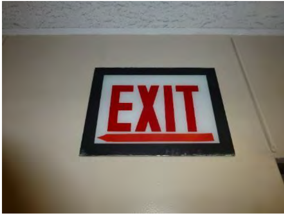
Figure 117. Non-illuminated exit sign
