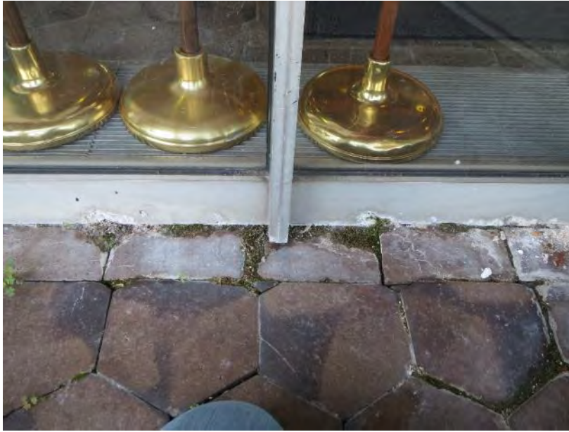
Figure 56. Missing fillet sealant in the joint between base of window wall and pavers. Note the significant organic growth and efflorescence.
