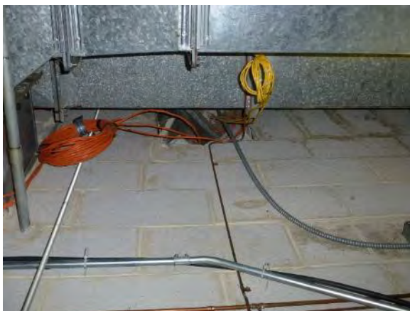
Figure 111. Unsealed penetrations in generator room
