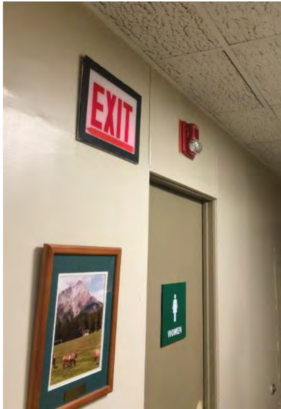
Figure 135. Exit signs and fire alarm notifiers (typical)
