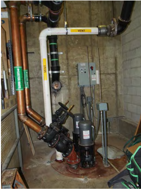
Figure 147. Sewage ejector pumps
