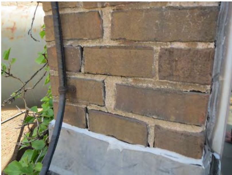
Figure 25. View of cracked and debonded mortar joints at the masonry piers at the north and east ends of the clerestory windows
