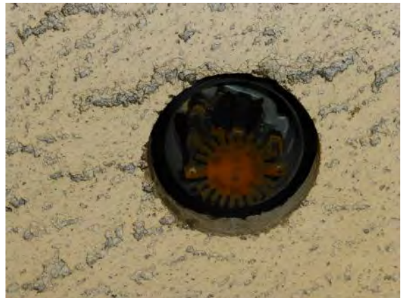
Figure 127. Concealed sprinkler without concealed cover plate
