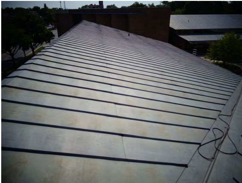
Figure 73. Bands of red discoloration on the surface of the standing seam panels on the upper roof on the east side of the building
