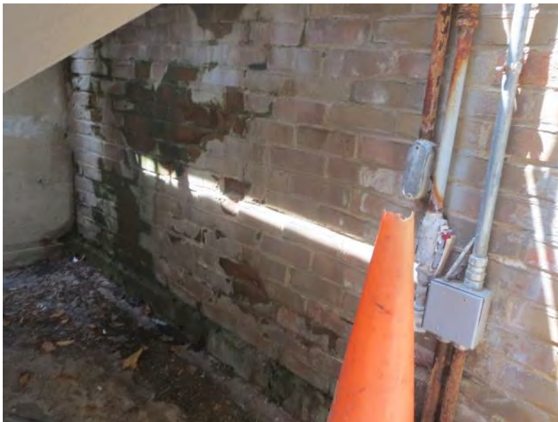
Figure 39. Moisture and efflorescence at the masonry cladding of the elevated plaza below the concrete stairs
