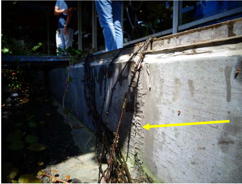
Figure 102. Close up view of open vertical solder seam in gutter liner. Note the plant growth and significant debris.
