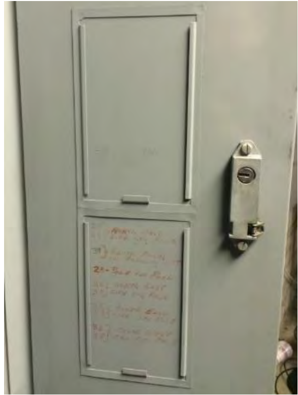
Figure 138. Panel schedules missing
