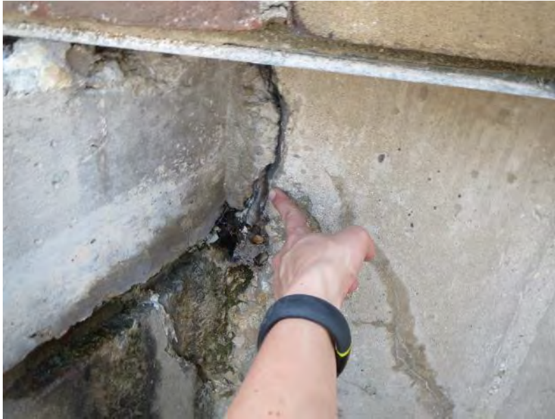
Figure 34. Moisture, biological growth and efflorescence at the crack at the concrete foundation wall
