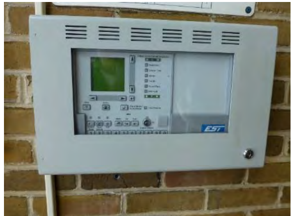
Figure 120. Fire alarm control panel in south lobby
