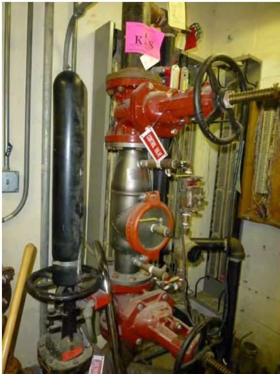
Figure 122. Wet-pipe sprinkler system riser
