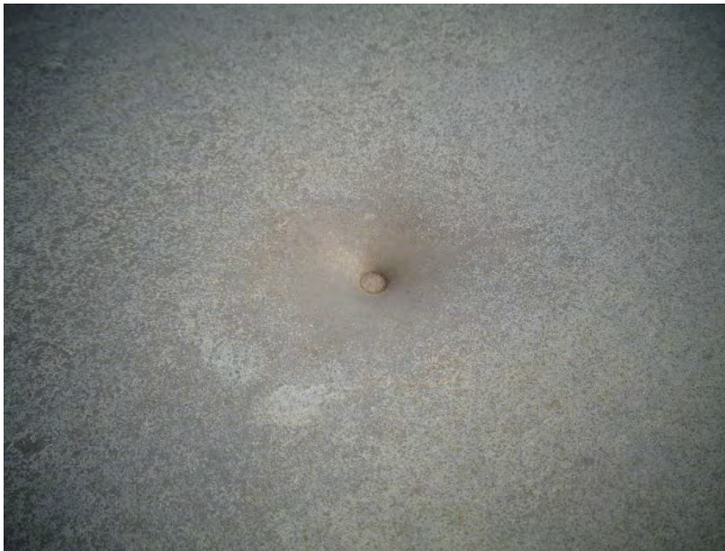
Figure 75. Typical impact damage at sheet metal roofing
