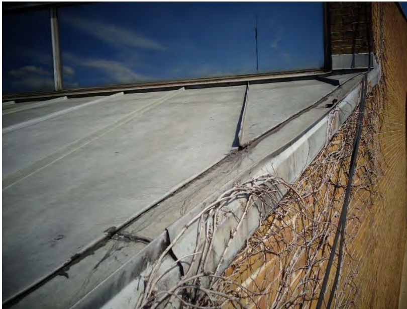
Figure 91. Rake-style edge metal at end wall
