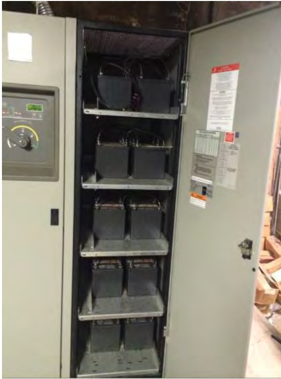
Figure 137. UPS batteries to be maintained or replaced regularly according to manufacturer's recommendations.
