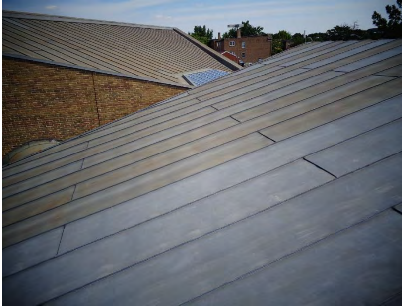
Figure 74. Consistently discolored panels at the north end of the upper roof on the east side of the building and on the Council Chamber annex (background)
