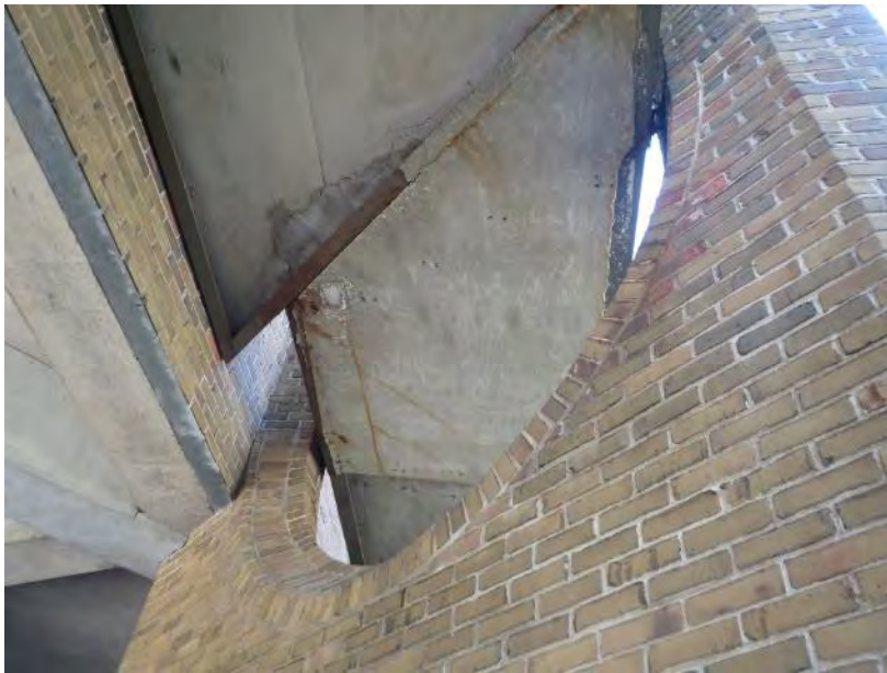
Figure 45. View of incipient spalls and corrosion of steel support at underside of the slab elevated ramped walkway at the Council Chambers Annex
