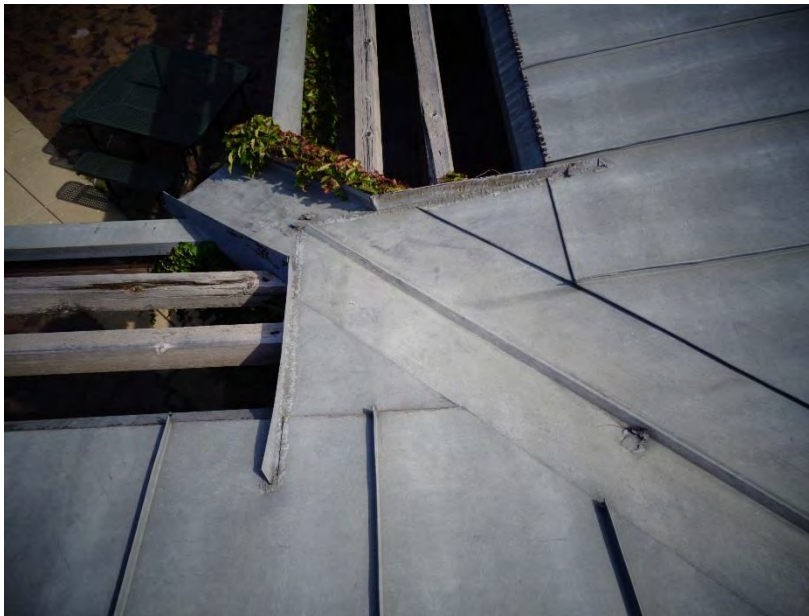
Figure 89. The valleys extend into sheet metal pans to carry the runoff water past the wood trellis
