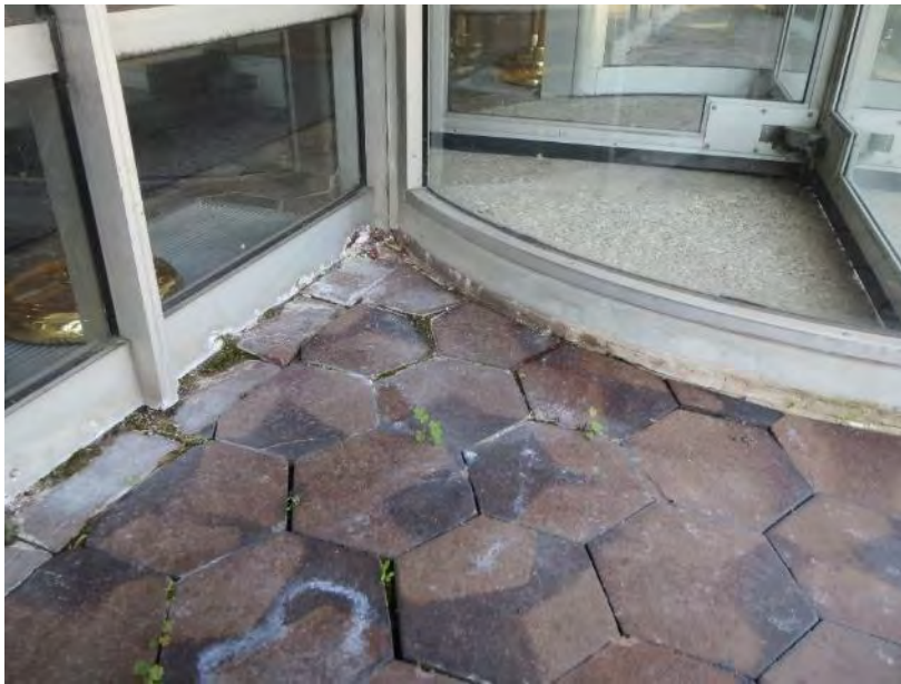
Figure 55. Missing fillet sealant in the joint between base of window wall and pavers. Note the significant organic growth and efflorescence.
