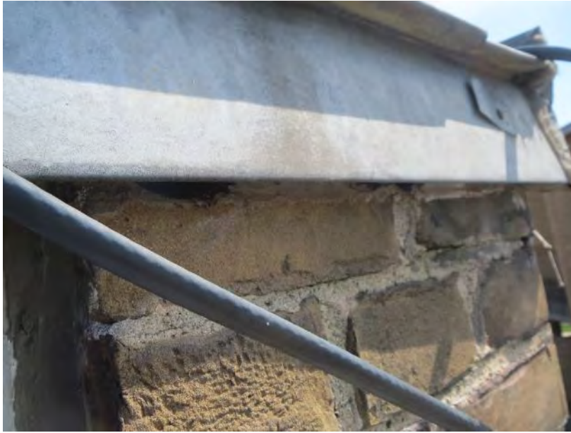
Figure 28. Voids exist between the top of the masonry pier and the roofing termination
