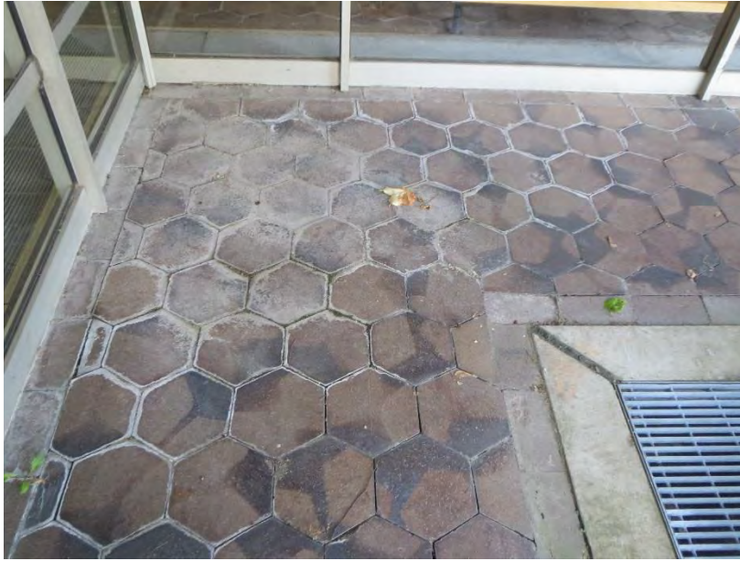
Figure 100. Efflorescence at joints between pavers at the window wall side of the gutter
