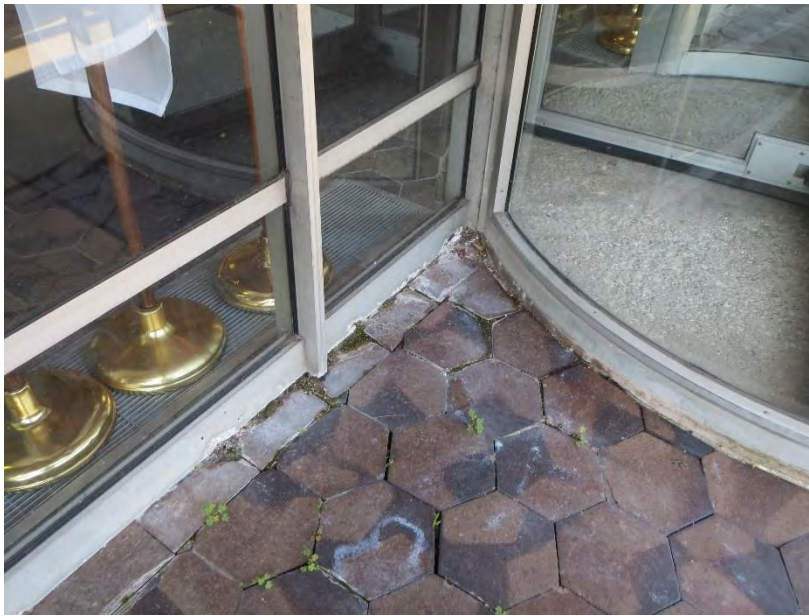
Figure 97. Displaced pavers and organic growth at joints between pavers near revolving door at south portion of plaza
