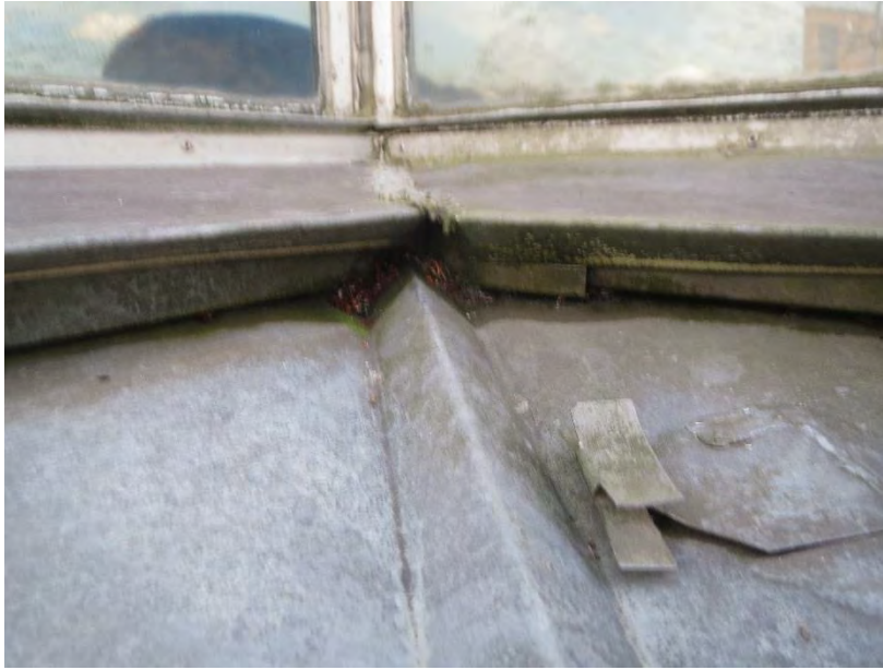
Figure 88. Water and debris were typically observed under the roof-to-wall closer at the top of the valleys
