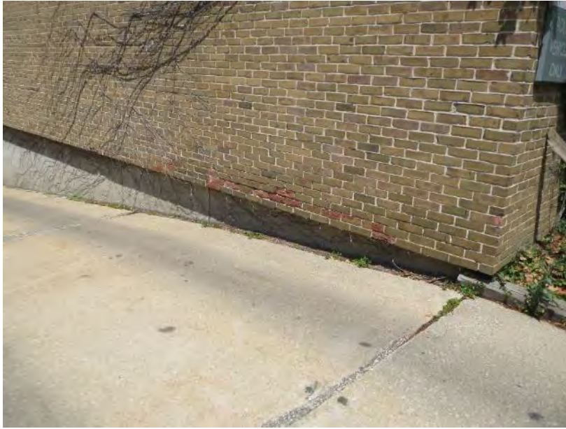
Figure 32. Face spalling of brick masonry above the shelf angle at the east end of the south facade
