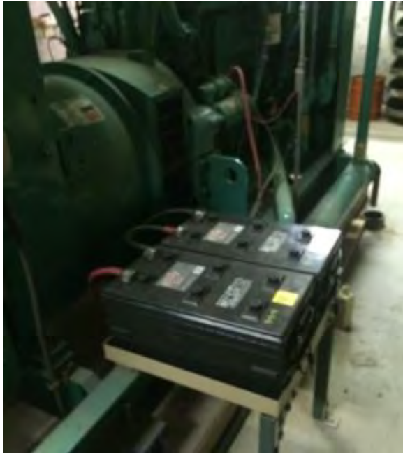
Figure 131. Close up view of generator batteries
