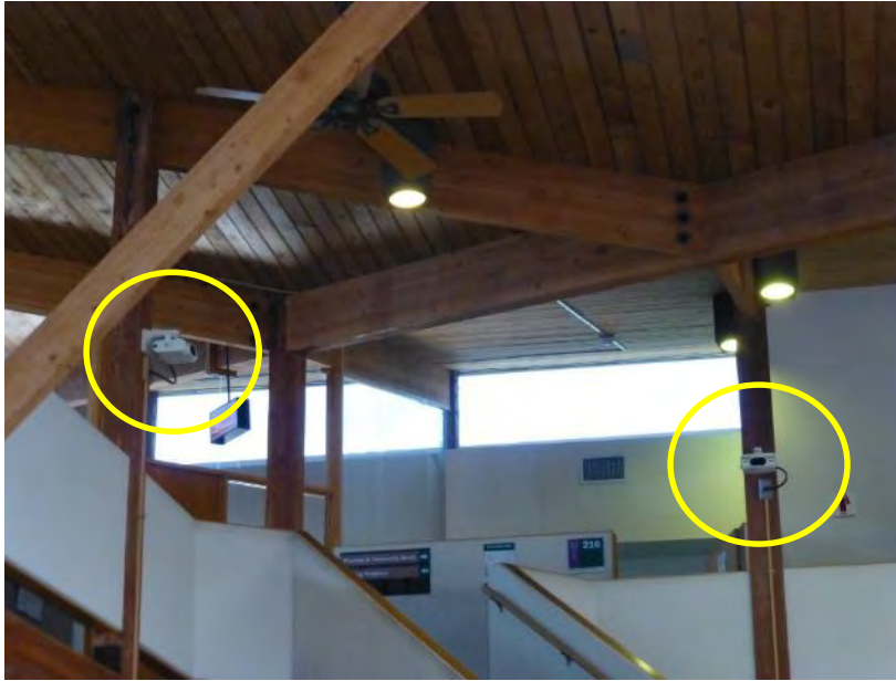
Figure 121. Beam-type smoke detectors
