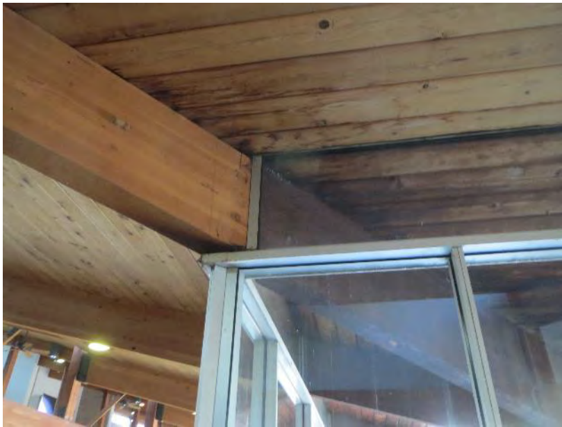
Figure 61. Water staining at underside of wood deck at the valley member above the window wall
