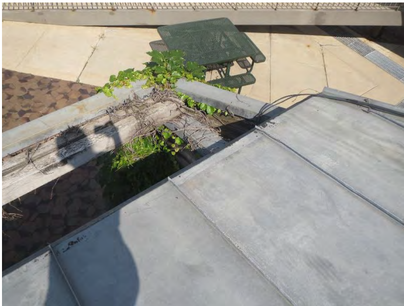
Figure 93. View of low slop roof edge and wood framed sunshade. Note how some of the wood framing is clad with sheet metal and significant vine growth.
