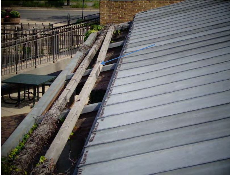
Figure 92. The end rafter of the wood sunshade is not adequately fastened and has displaced.
