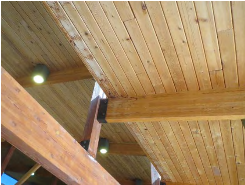
Figure 65. Water staining at the wood decking under the clerestory windows at the east side of the plaza
