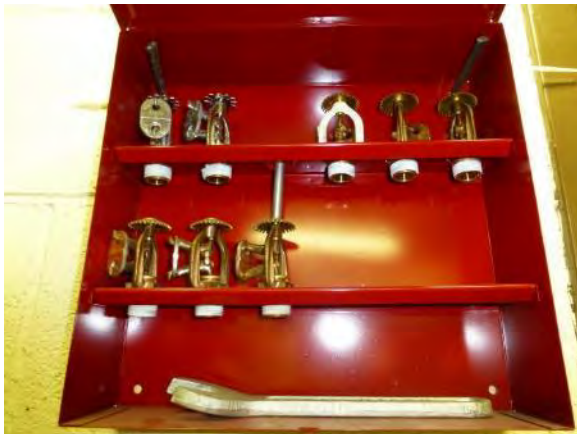
Figure 126. Spare sprinkler cabinet
