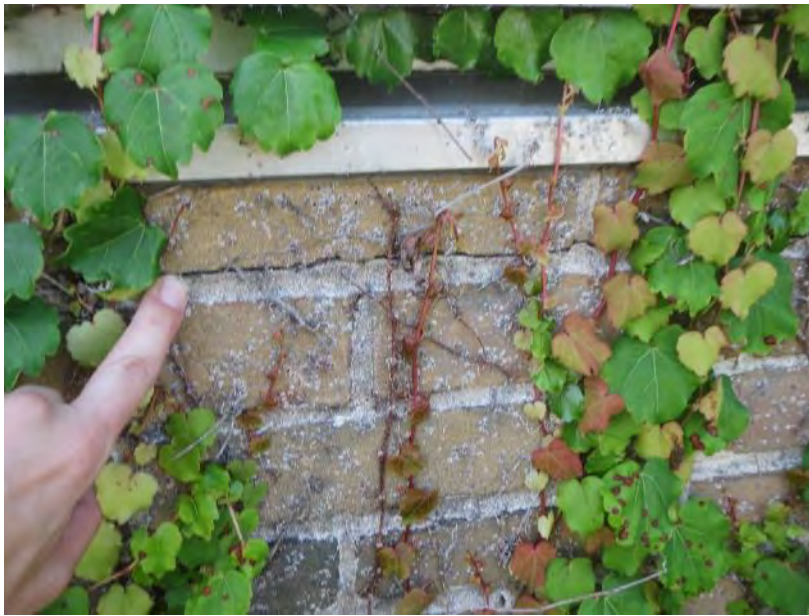
Figure 31. Typical cracked and debonded mortar joints
