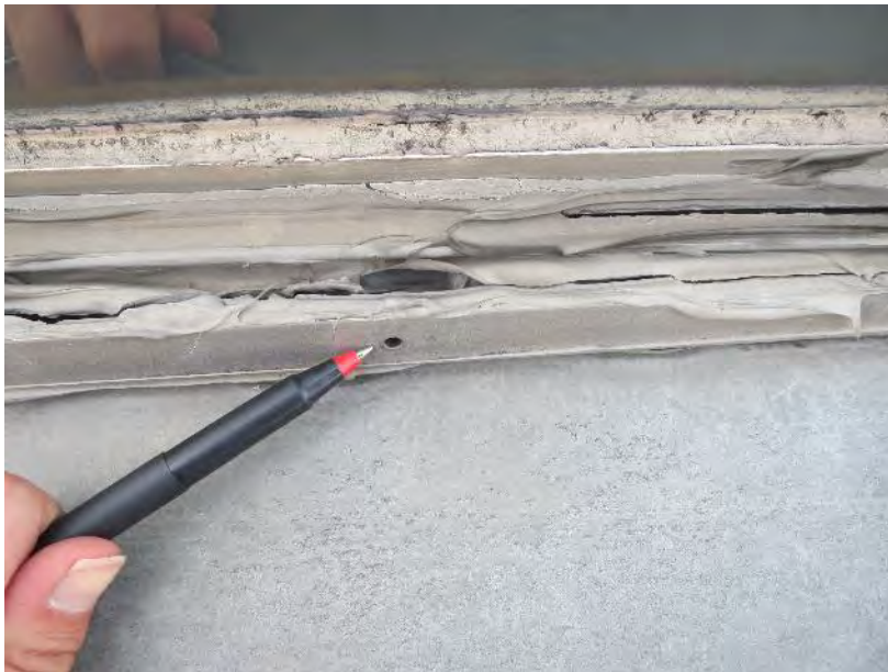
Figure 53. Missing fasteners and severely debonded sealant at the counterflashing at the base of the clerestory windows
