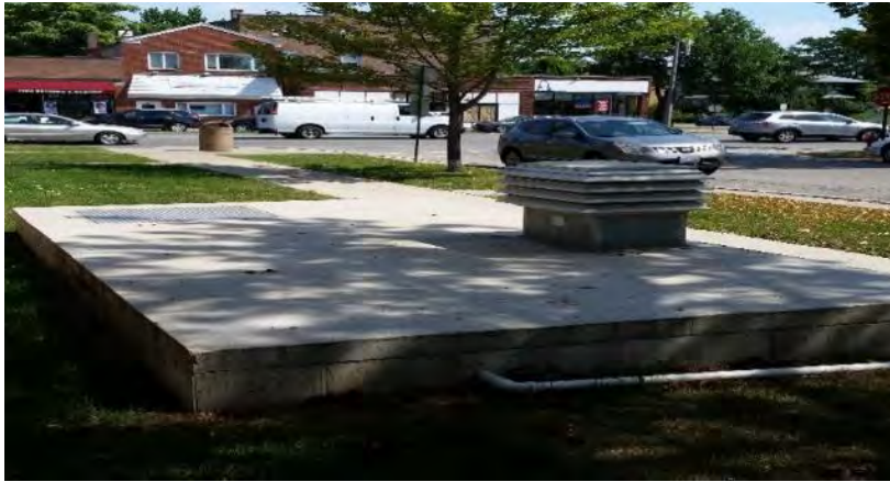
Figure 145. S-6 geothermal vault mounted heat pump
