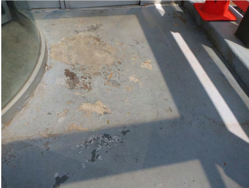
Figure 44. View of deteriorated traffic coating at the top side of the slab at the entrance bridge
