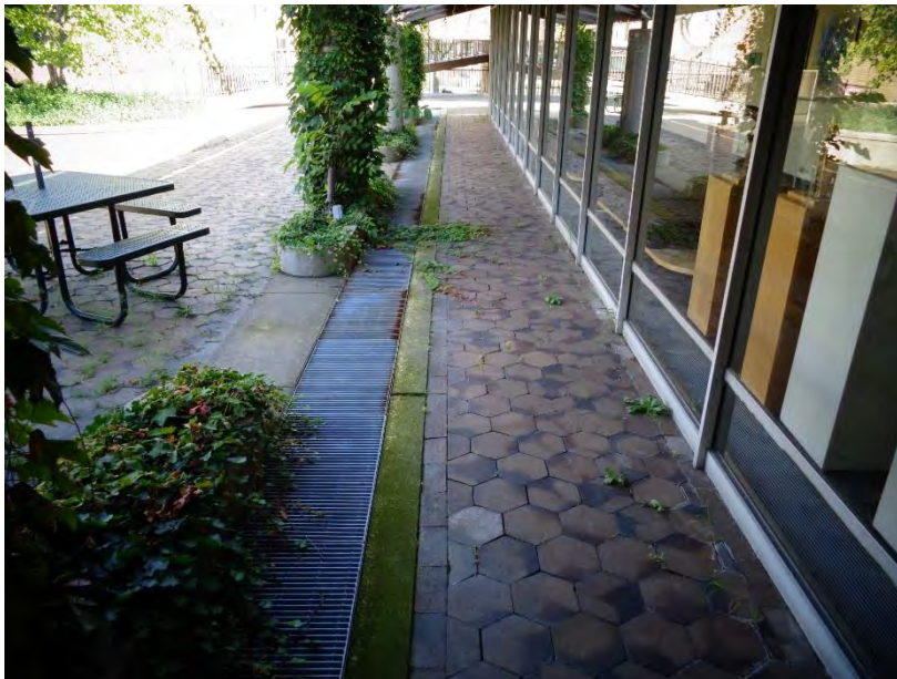
Figure 99. Overall view perimeter gutter at plaza. Note the organic growth at the concrete gutter structure and ivy at the sunshade support structure.
