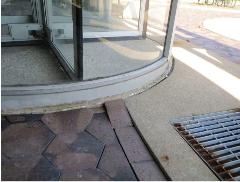
Figure 98. Displacement of pavers at concrete curb at revolving door at south side of plaza
