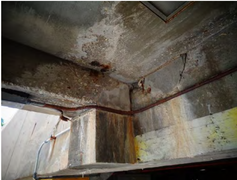
Figure 43. View of incipient spalls and corrosion of steel reinforcing bars at underside of the slab elevated entrance bridge at south facade
