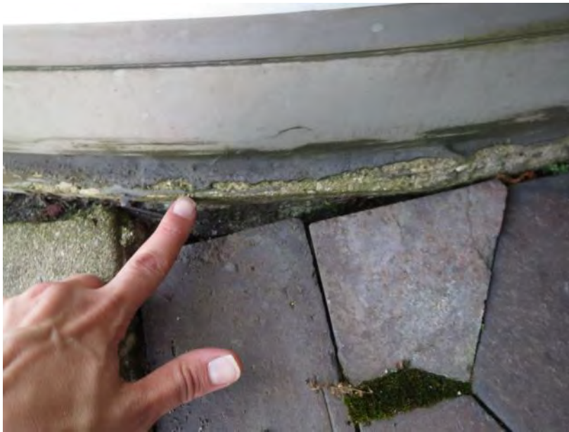
Figure 57. Deteriorated sealant at the joint between the concrete curb and the base of revolving door. Note displacement of pavers and organic growth at pavers at revolving door curb.
