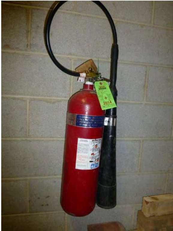
Figure 128. Fire extinguisher with current inspection tag
