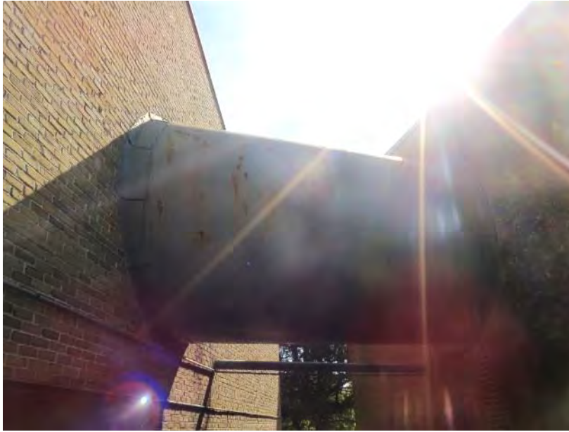
Figure 46. Surface corrosion at the painted steel tube connecting link between the council chambers annex and the main Village Hall building
