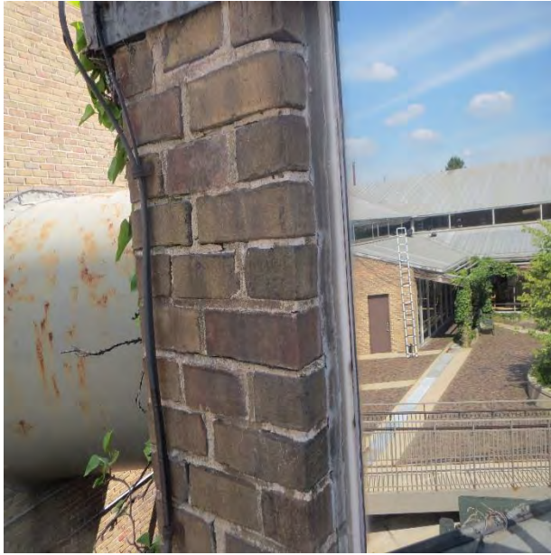
Figure 26. View of cracked and debonded mortar joints at the masonry piers at the north and east ends of the clerestory windows
