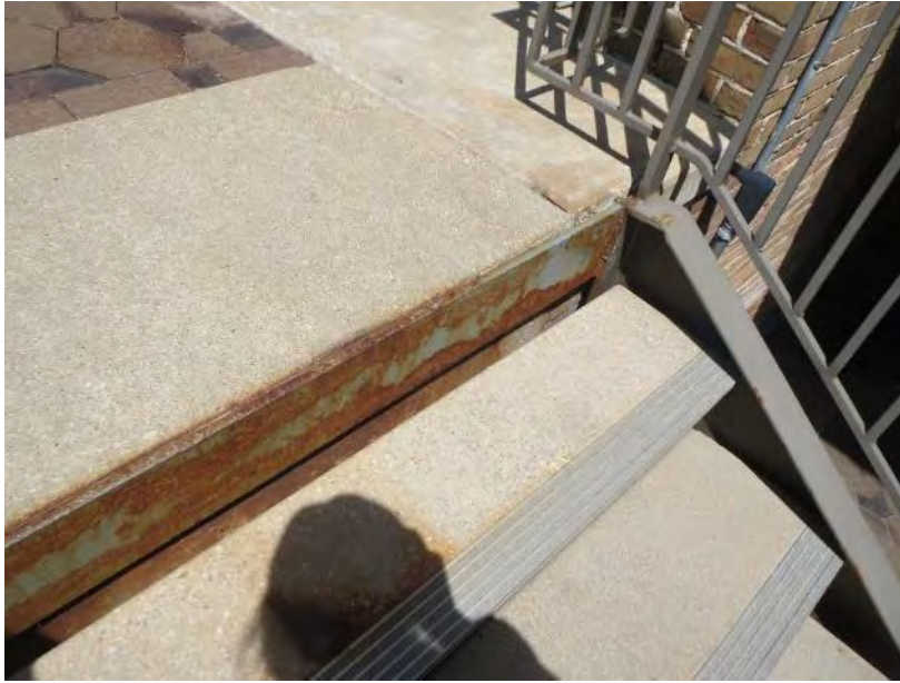
Figure 40. Corrosion scaling at the metal panning of the stairs between the elevated plaza level and the original reflecting pool plaza area
