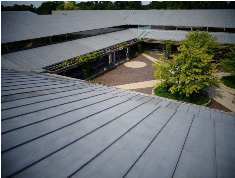
Figure 69. Close up view of the low slope upper standing seam metal roof
