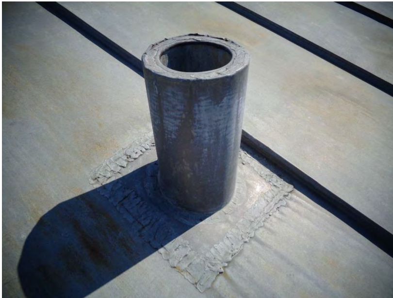
Figure 77. Vent stack flashing
