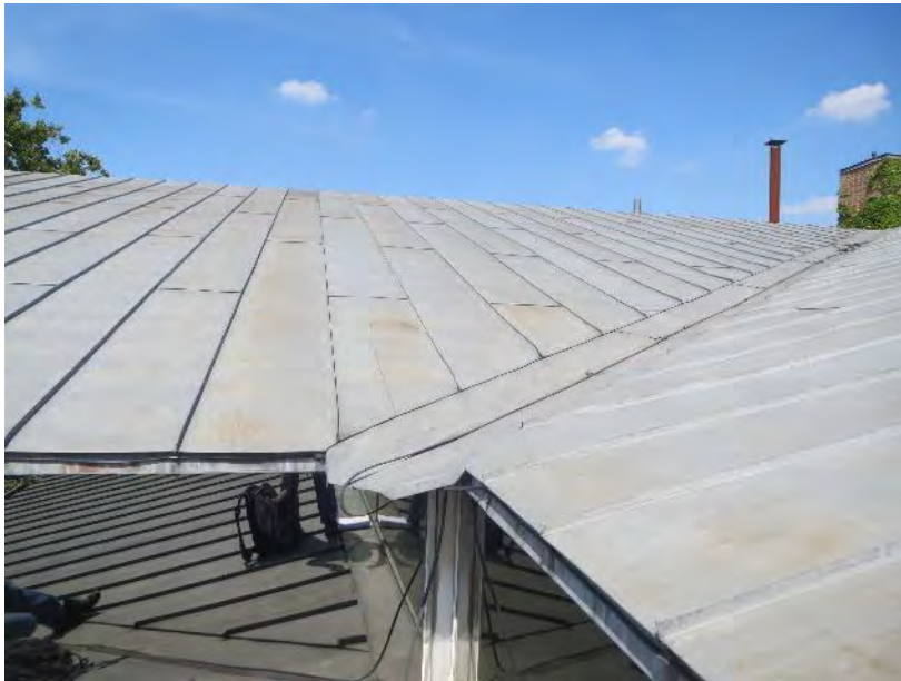
Figure 71. Close up view of typical valley configuration of the upper low slope roof above the clerestory windows
