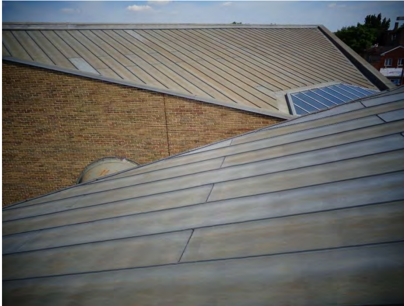
Figure 70. View of the standing seam metal roof and skylight above the Council Chambers Annex
