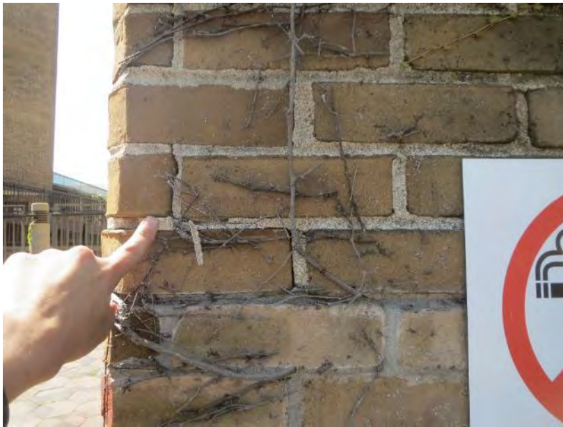
Figure 29. Typical cracked and debonded mortar joints
