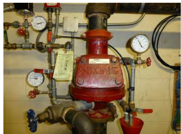
Figure 123. Dry-pipe sprinkler system riser
