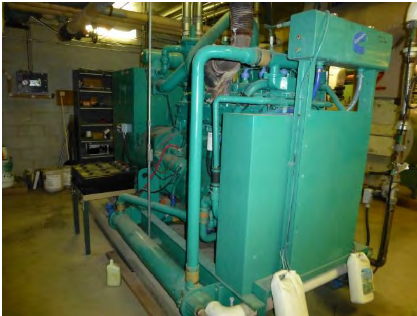
Figure 130. Emergency generator
