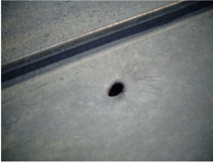
Figure 76. Small hole (approximately 1/2 inch) diameter at the west portion of the sheet metal roofing
