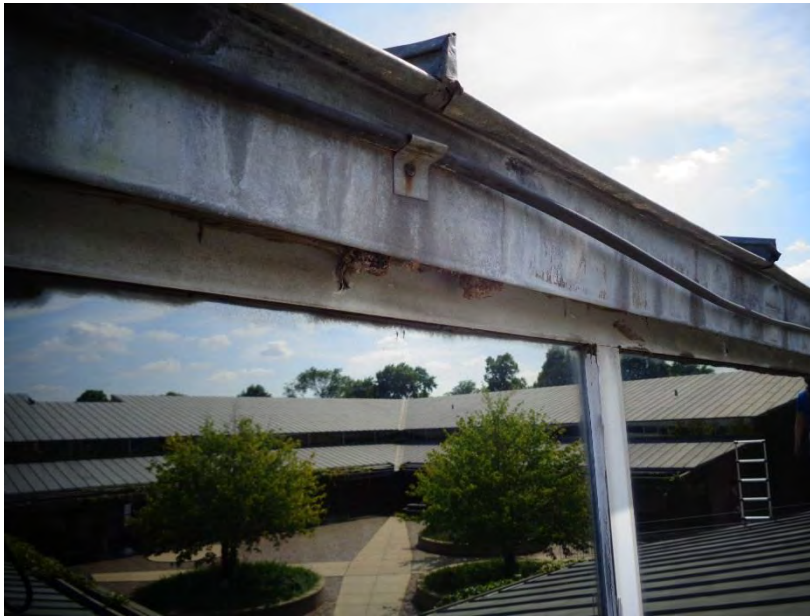
Figure 81. Close up of edge metal above top of clerestory windows
