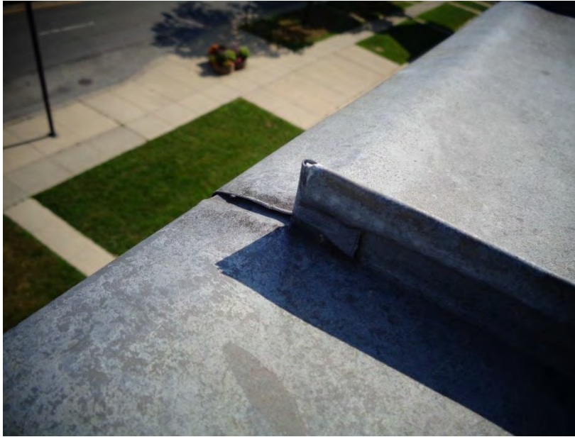
Figure 80. Close-up of cut and folded standing seam at the top of the upper roof level
