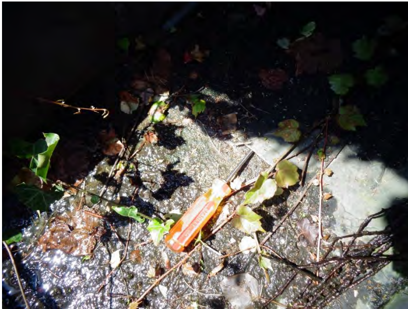
Figure 103. Close up view of open horizontal lap seam in gutter liner. Note the plant growth and significant debris.
