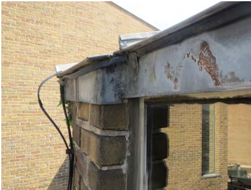
Figure 27. Counterflashing/ roof termination at the masonry piers and the top of the clerestory windows
