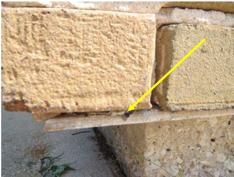
Figure 21. Close up view of brick at steel shelf angle. Note the flashing on the shelf angle.
