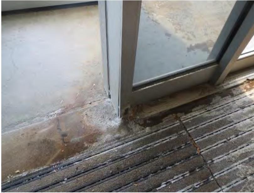
Figure 60. Efflorescence, surface corrosion and staining at base of storefront at south entrance
