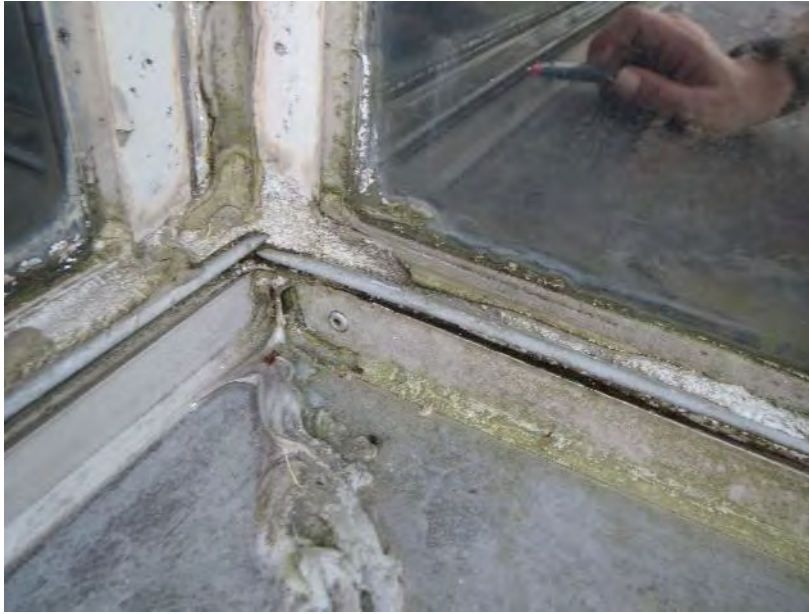
Figure 52. Crazed sealant at counterflashing at the base of the clerestory windows and deteriorated gaskets/wet seals at the metal to glass joints at the clerestory windows at a valley location
