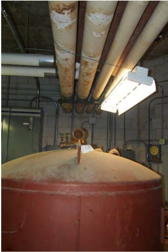
Figure 149. Pipe corrosion and deterioration of insulation
