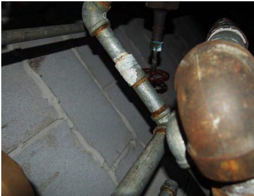
Figure 148. Pipe corrosion
