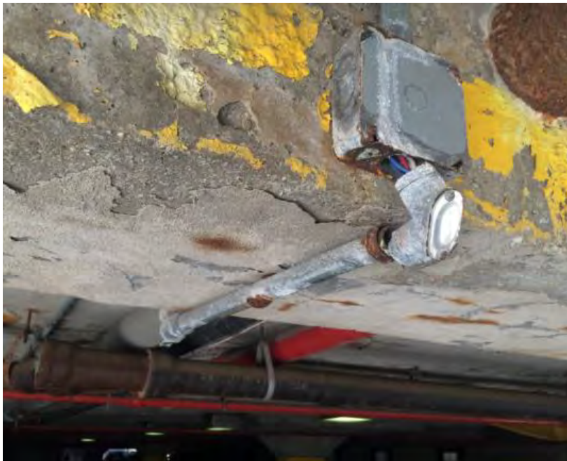
Figure 134. Underground parking structure lighting conduits (damaged)
