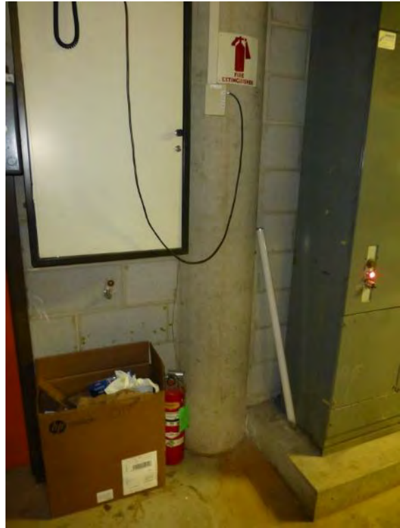
Figure 129. Fire extinguisher on floor outside generator room
