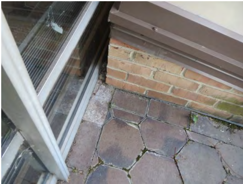
Figure 59. Deteriorated sealant at the joint between the concrete curb and the base of skylight. Note displacement of pavers and organic growth at pavers at skylight.
