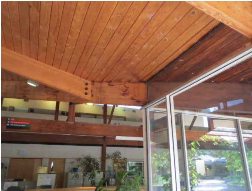
Figure 63. Water staining at the valley member above the window wall. Previous water infiltration has been reported at the valley members.
