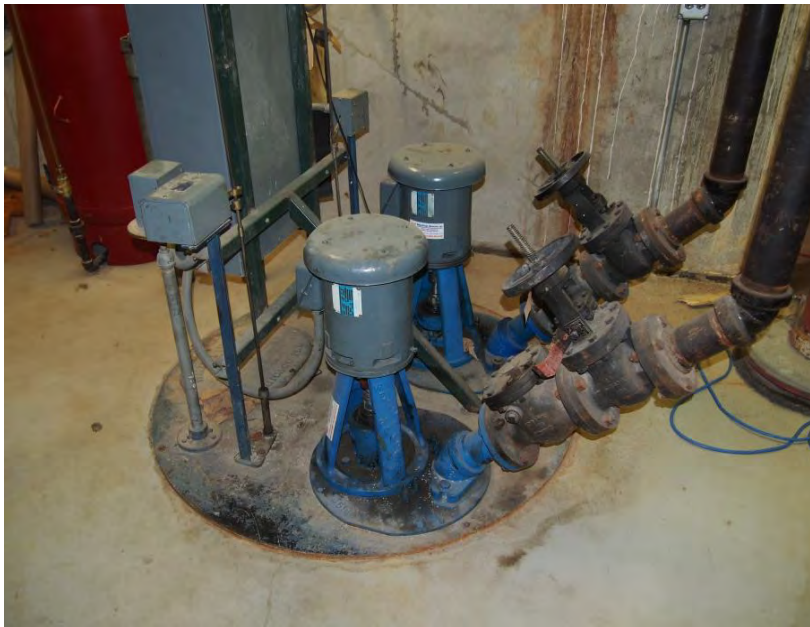
Figure 146. Existing sump pump system
