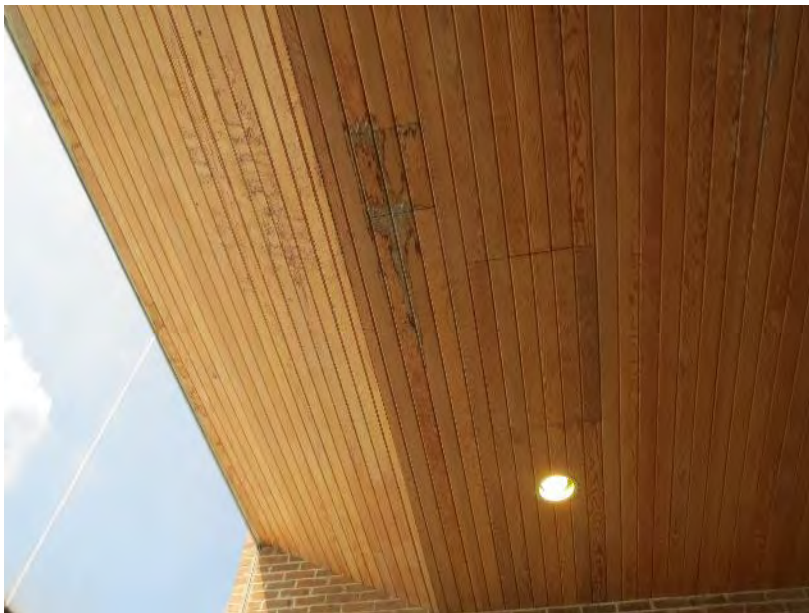
Figure 67. Water staining at the underside of wood decking below the flat roof portion of the building above the south entrance
