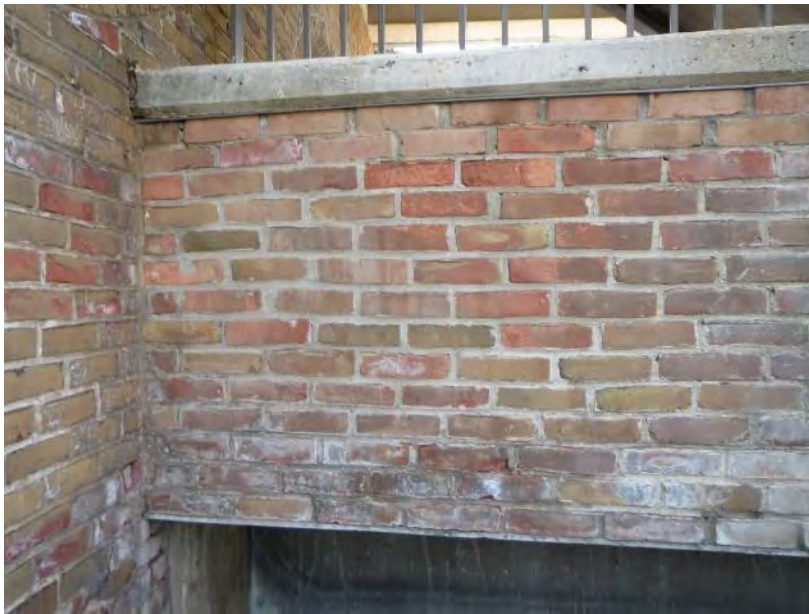
Figure 37. View of efflorescence at the brick cladding at the edge of the elevated plaza level
