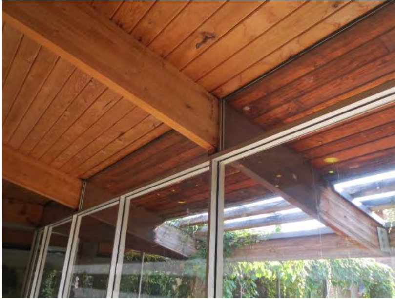
Figure 62. Water staining at underside of wood deck at typical rafters above the window wall
