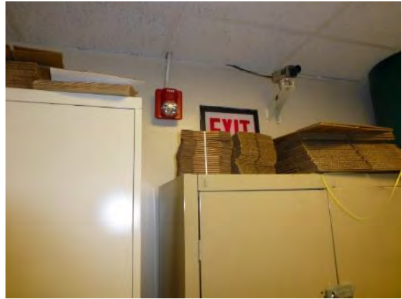
Figure 118. Exit sign obstructed by storage
