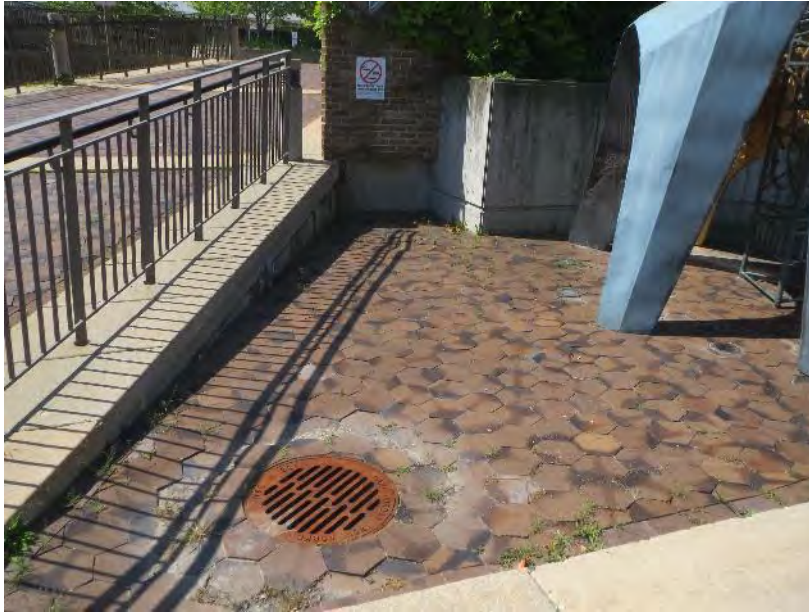
Figure 96. View displaced pavers at area drain
