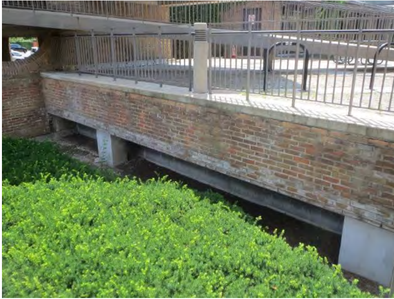
Figure 36. View of efflorescence at the brick cladding at the edge of the elevated plaza level
