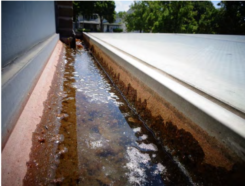
Figure 95. Standing water at gutter between the building wall at the glass canopy above the south entrance walkway
