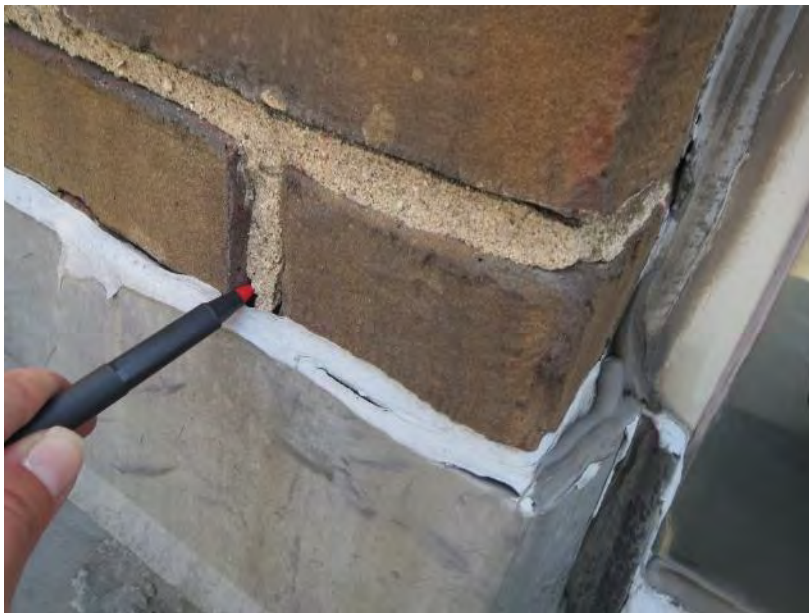
Figure 87. Debonded, crazed and split sealant at the roof counterflashing at the base of the masonry pier
