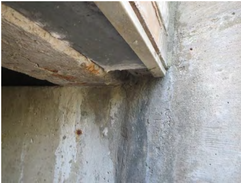
Figure 41. Spalling and efflorescence at steel angle at concrete beam at the ramped walkway
