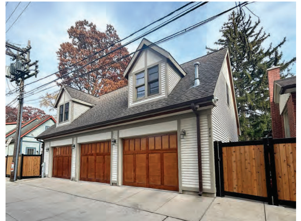
View from alley looking northeast at Erie garage
