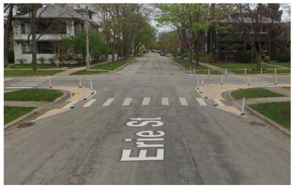
Figure 5. Paint and Post Curb Extension Example
