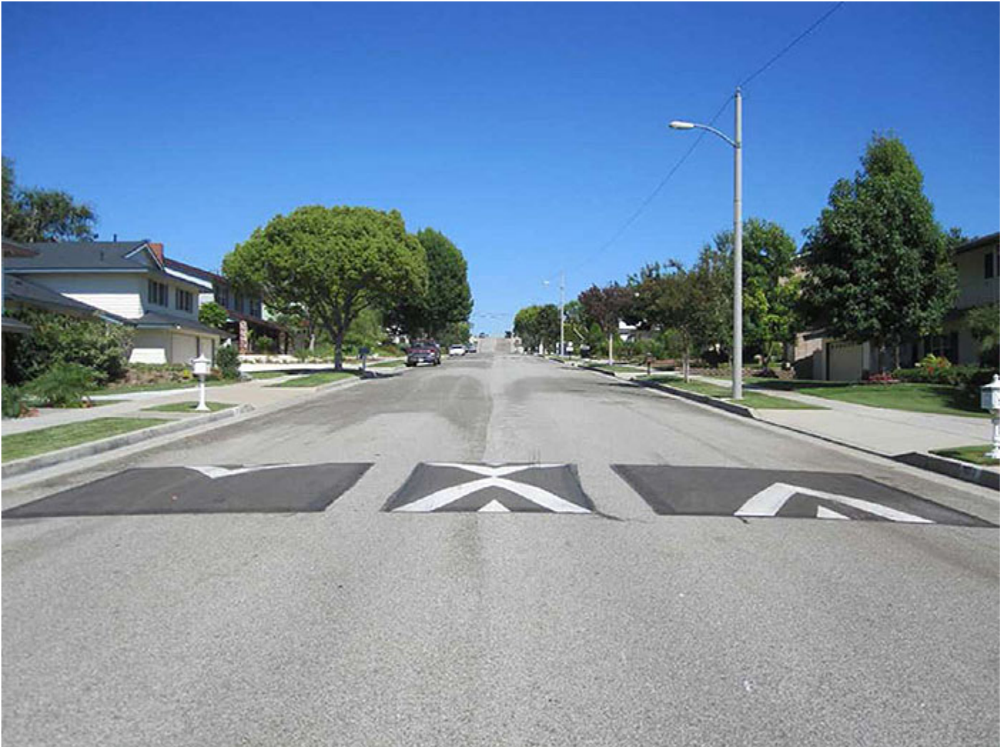
Figure 6. Speed Cushion Example
