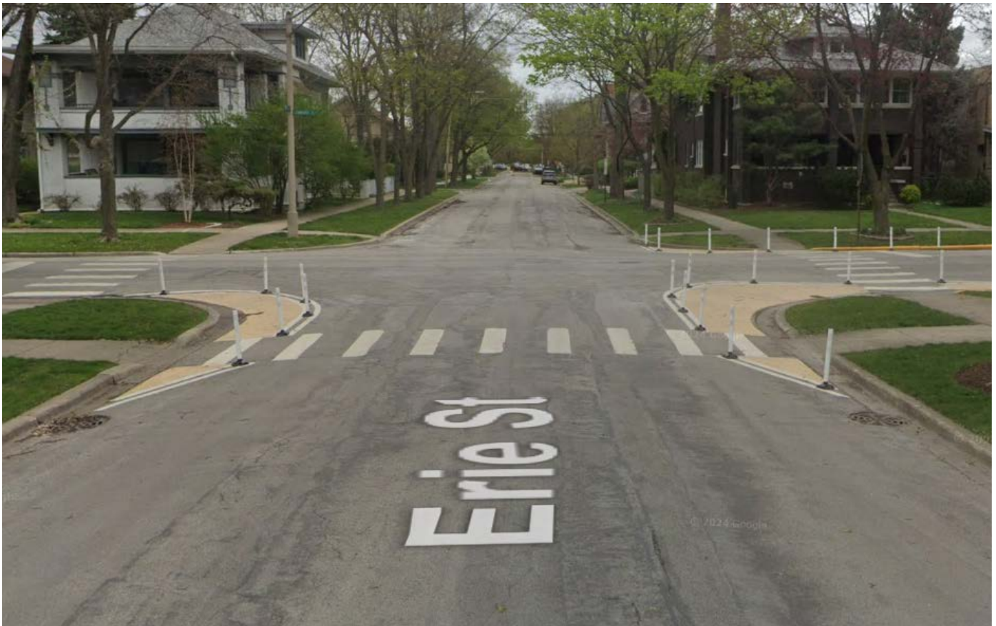
Image 1. Paint and Post Curb Extension Example
