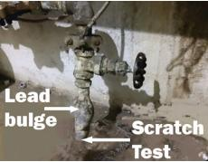
The public side of water services, being the portion between the Village's water main and the homeowner's water shut-off valve, will be upgraded from lead or galvanized iron pipe to copper whenever the water main is replaced or if the homeowner elects to replace the private side of their water service.
