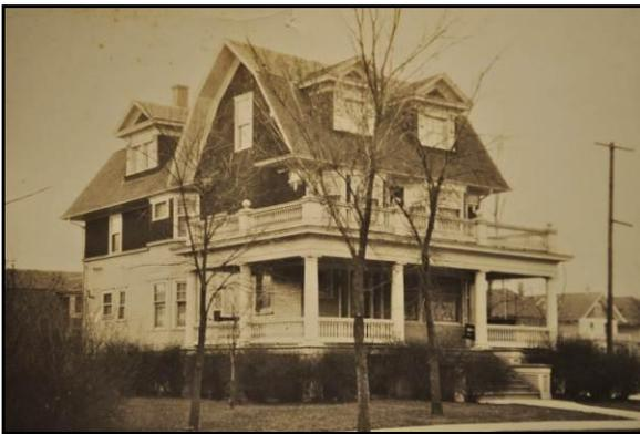
Historic photos were also vital in the design and reconstruction of the original open front porch. All of the wood siding and wood shingles were repaired or replaced as needed, stripped and repainted.
