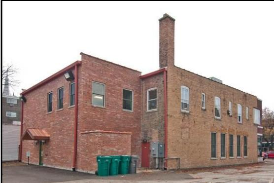
The project preserved the exterior terra cotta and brick façade. A rear addition made the building ADA accessible and allowed for the repair and restoration of the historic interior second-floor offices.
