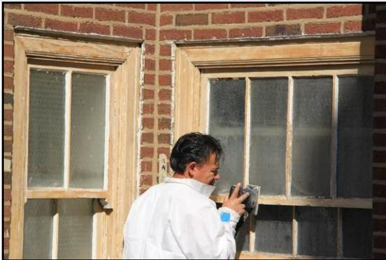
The Condo Board hired **Historic Home and Window Restoration** out of Aurora to begin a window restoration project in the fall of 2011. The windows were in good physical condition, but needed repairs to the glazing putty, sills, and trim. In addition to repainting, the contractor also replaced weatherstripping and broken sash cords, which improved the overall ease of operation and thermal efficiency.
