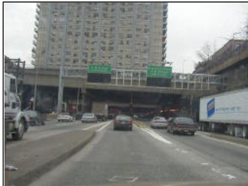
Originally constructed as a two-lane bypass, the expressway now carries more than 250,000 vehicles per day on its 12 lanes of roadway. The original 178th Street and 179th Street tunnels were designed in traditional Moses-style, utilizing stone-faced arch portals and "Whitestone" lightposts. Viaducts with single circular supports that connected the tunnels with the Washington (Heights) Bridge are still in use today.
