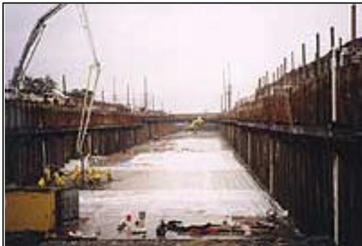
The tunnel parallels a canal where the excavation ranged between 10 and 35 feet deep and extended into loose silty sands, 30 feet below the water table. The work included the design of the sheeting, high capacity tiebacks, and a jet grout wale and strut system to support the sheeting at subgrade. Design of the excavation support includes a 45-foot deep pump station.
