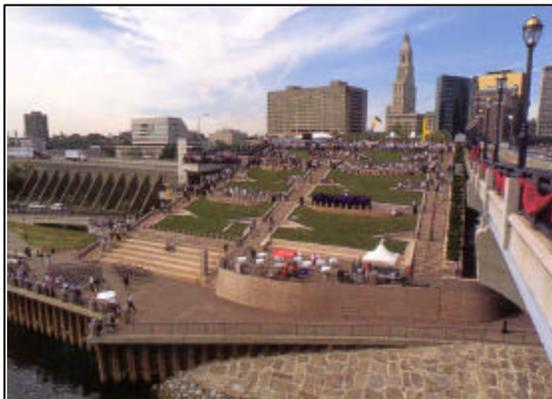
Restoration of pedestrian access to the riverfront required lowering the 1-91 southbound viaduct to grade while maintaining traffic flow. This permitted the construction of the elevated 1.5-acre landscaped deck (Riverfront Plaza) that spans 1-91, the railroad, and the flood control walls, and includes a landscaped, platform-supported, terraced structure that steps down to the riverfront. A pedestrian and bicycle pathway over the river was incorporated into the Founders Bridge reconstruction.
