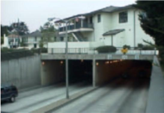
**Fig. 3a:** Lighthouse Ave. Tunnel – has extensive pumping / collection storm water system due to below sea level
