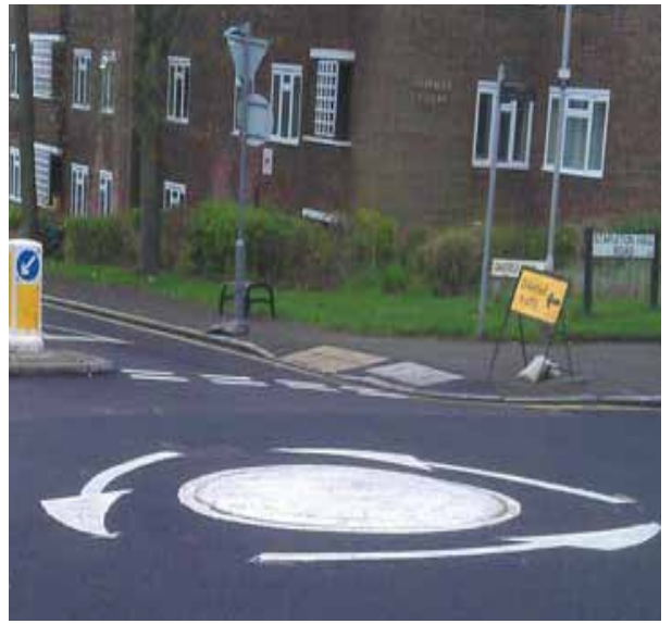
PAINTED MINI ROUNDABOUTS May be used prior to permanent installation, though they are not as effective. Photo credit: http://www.lbc.co.uk/
