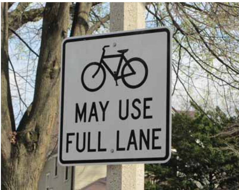
BIKES MAY USE FULL LANE SIGN (R4-11) Install together with pavement markings along Neighborhood Greenways routes.
