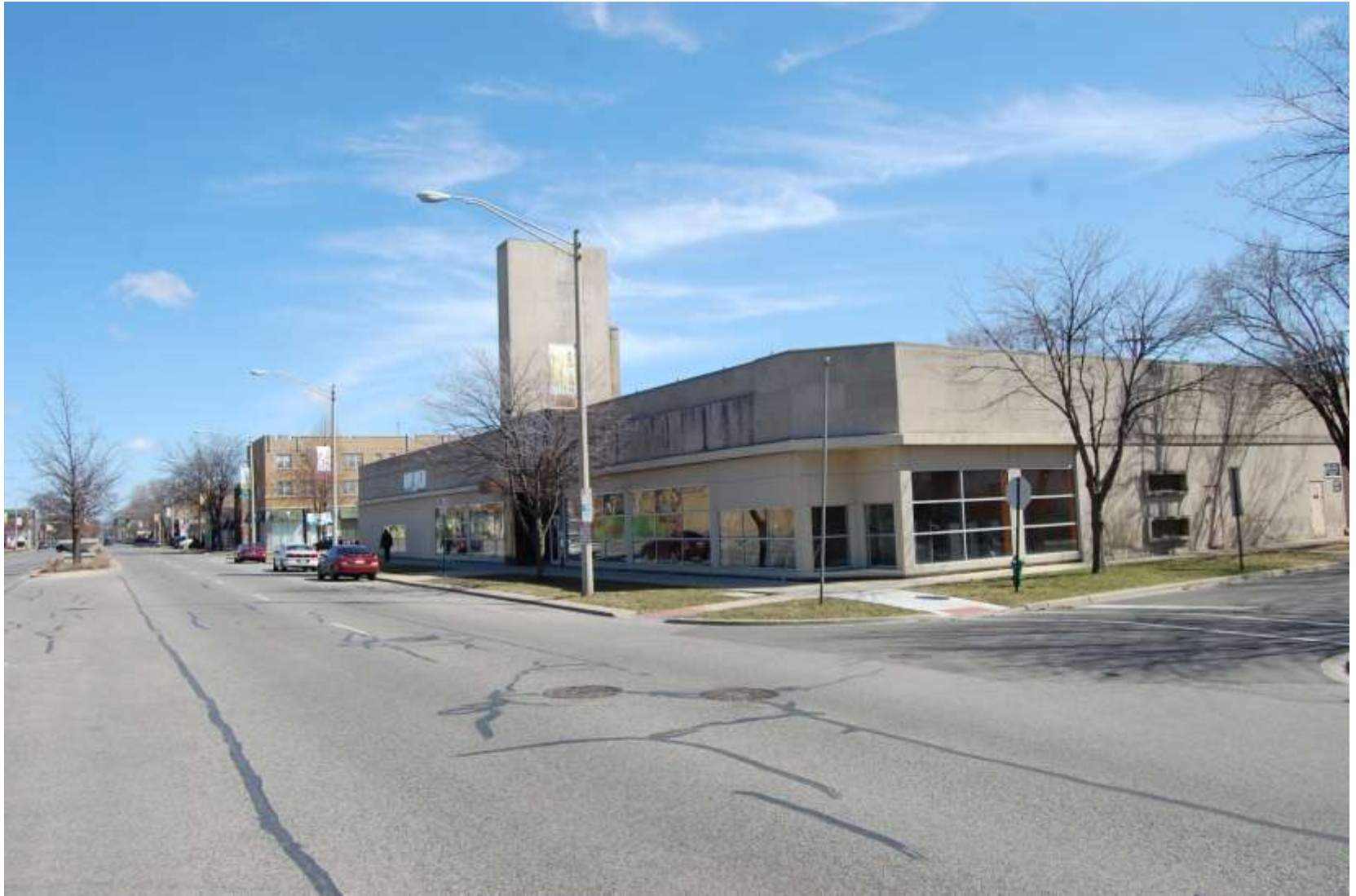
Madison at Euclid—Existing Conditions
