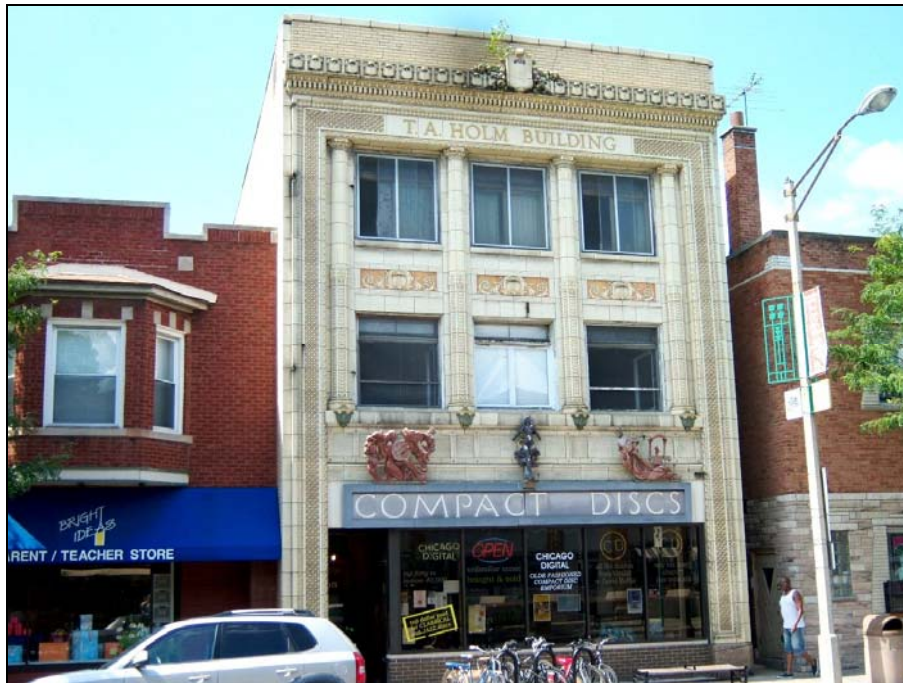
T. A. Holm Building, 905 S. Oak Park Avenue
