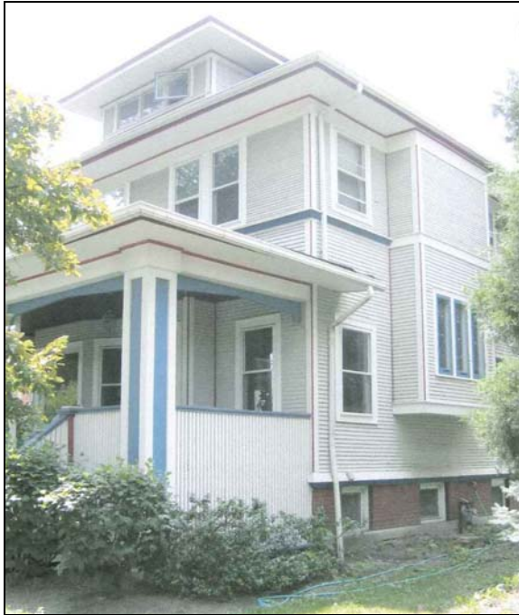
Front and north facades showing side rails of porch and art glass casement windows in bay
