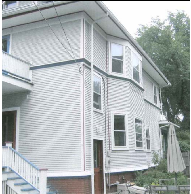
South façade looking Northeast
