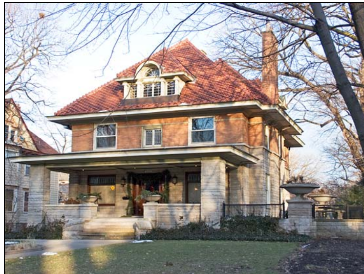
422 Forest Avenue (1900) (Source: Village of Oak Park)
