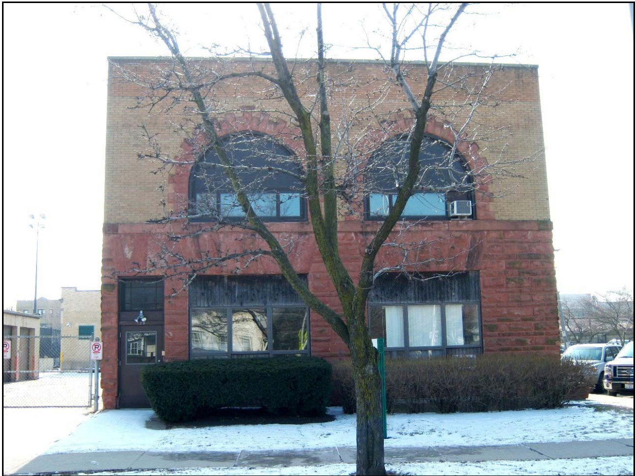
Cicero Fire House No. 2 129 Lake Street
