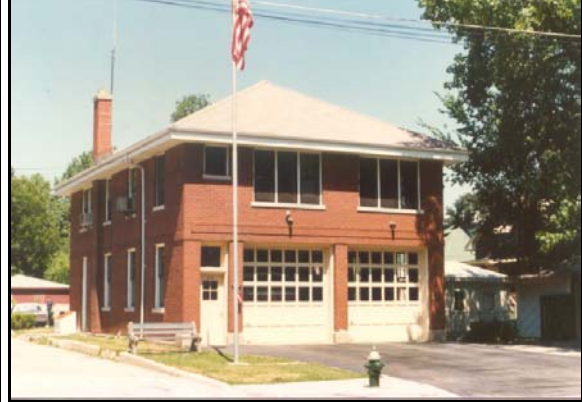
North Fire Station c. 1983
