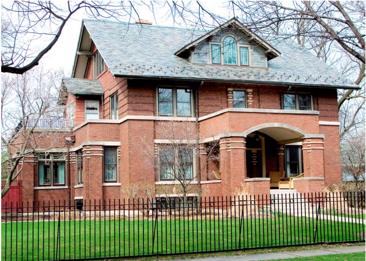
Vernon W. Skiff House 633 N. East Avenue
