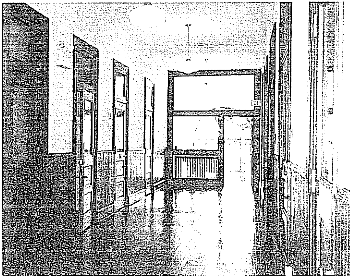
Two historic schools in York, Pa , were transformed into a low- to moderate-income 17 unit apartment complex using the historic rehabilitation tax credit. In order to comply with fire safety regulations while still retaining the school's historic character, the second floor hall was enclosed with custom-made wood and glass smoke barrier walls that allow a clear view of the round-arched windows at each end of the building
